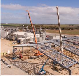
CRANE BEING USED TO REPLACE STRUCTURAL STEEL AND ROOFING
