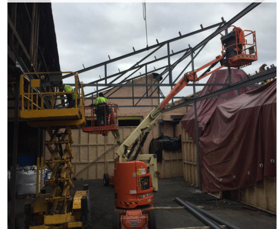
HOARDING AND TARPS SET UP TO PROTECT MACHINERY DURING REPAIRS
