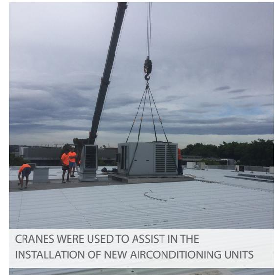
CRANES WERE USED TO ASSIST IN THE INSTALLATION OF NEW AIRCONDITIONING UNITS
