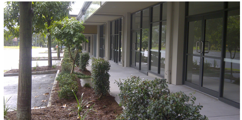
THE REPAIRED AND IMPROVED COMMUNITY HUB & SHOPPING VILLAGE BACK IN BUSINESS, MAY 2013
