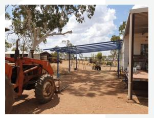
The purlins had to be lifted into place by forklift (yes the Graziers have all the tools). The purlins where welded in place, whilst a team chased spot fires below.
