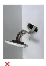
Electrician is to be engaged for the removal of General Purpose Outlets (GPO's). All other trades are not to handle, remove, or relocate GPO's. Contact Supervisor if an electrician is required.
