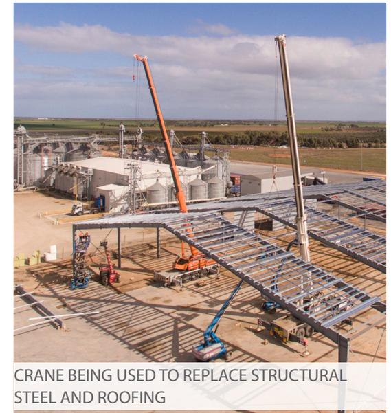
CRANE BEING USED TO REPLACE STRUCTURAL STEEL AND ROOFING
