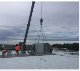
CRANES WERE USED TO ASSIST IN THE INSTALLATION OF NEW AIRCONDITIONING UNITS
